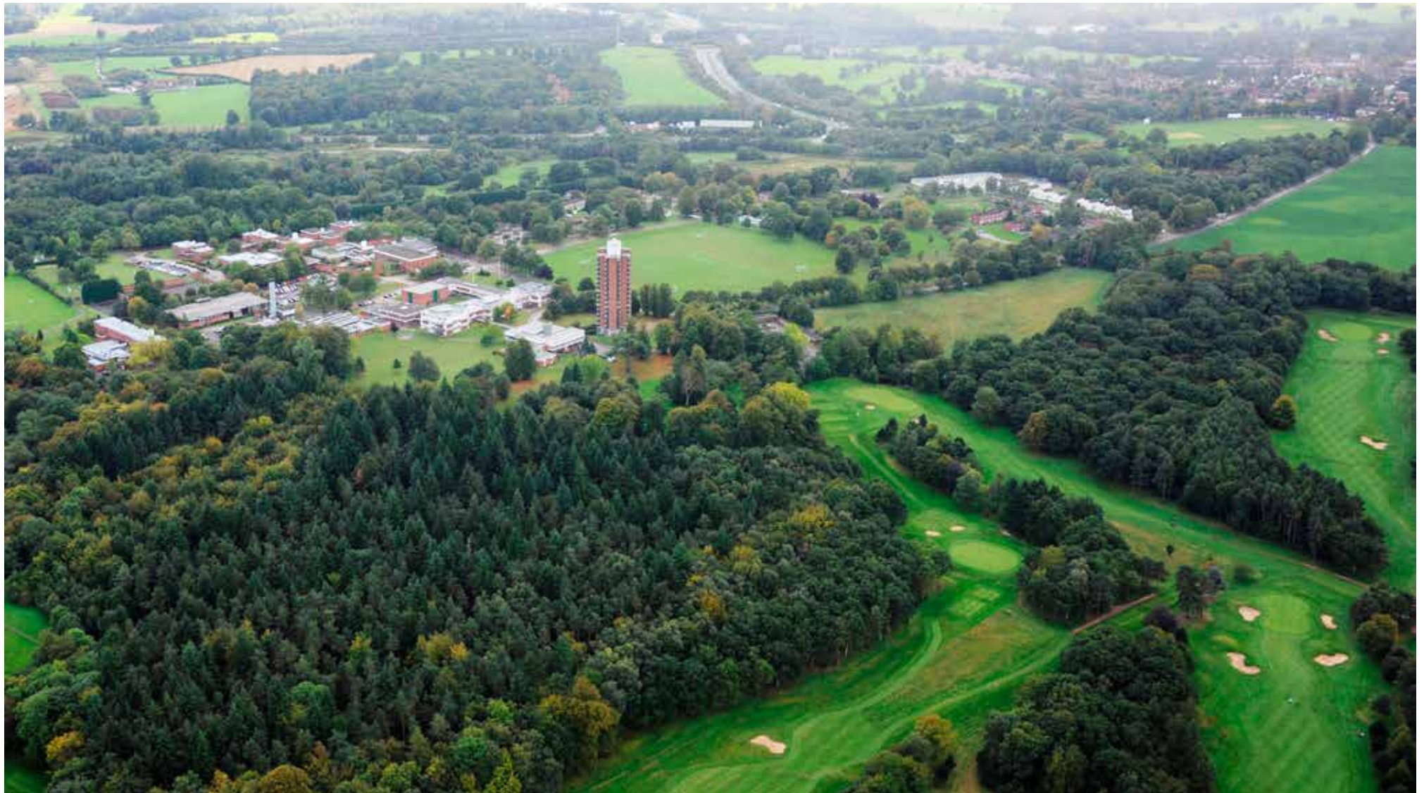
Aerial view of Wilton Park Opportunity Site
