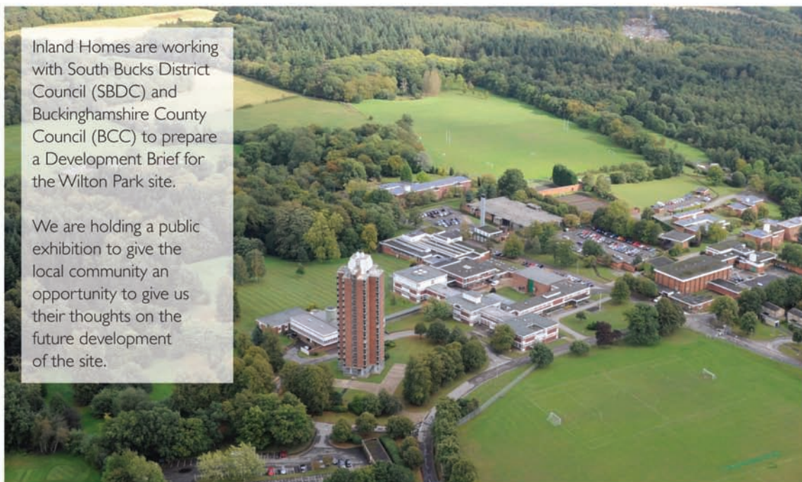
A view of the existing Wilton Park site
